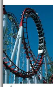
If the ride is propelled by gravity then the designer must make sure that the car has this minimum speed when it reaches the top.
