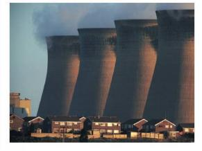
The overall efficiency of a coalfired power station is around 40% as not all of the chemical energy from the coal gets converted to electricity. The exhaust gases from the original burning take some of the heat, as does the heat given out when the steam from the turbine condenses. There is also some friction in the components of the turbine and generator.
