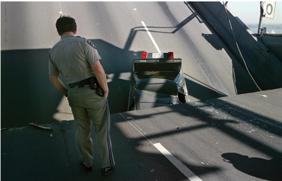
On 17 October 1989, an earthquake severely damaged the Bay Bridge, San Francisco, causing 68 deaths.
